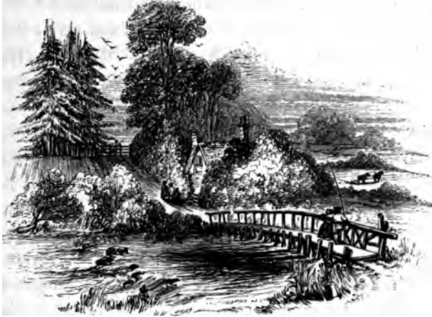
The Bridge over the Weare.
